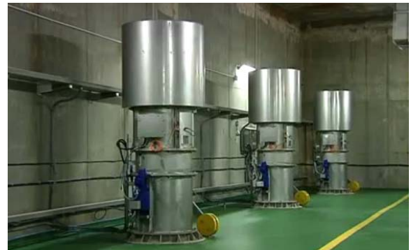
Fig. 1. Turbines in Mutriku MOWC breakwater
