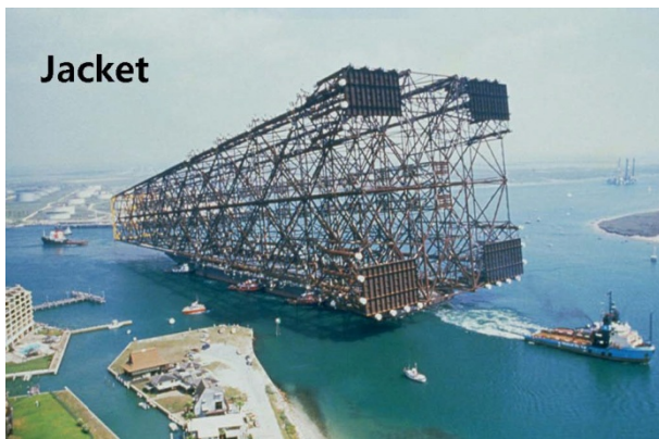
Fig. 1 Example of an underwater jacket structure.
