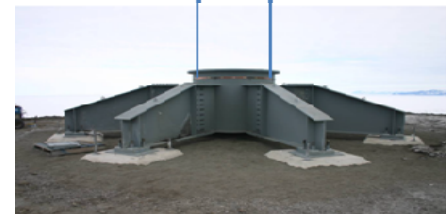
Fig. 6. Tidal turbine foundation using marine micropiles
