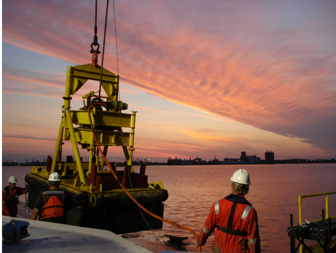
Fig. 7. Deploying a seabed CPT system from a barge in Norfolk, Virginia.
