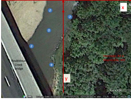
Fig. 14. Experiment spot for Field Test 3 at I-44 Roubidoux Creek Bridge, Waynesville, MO.
