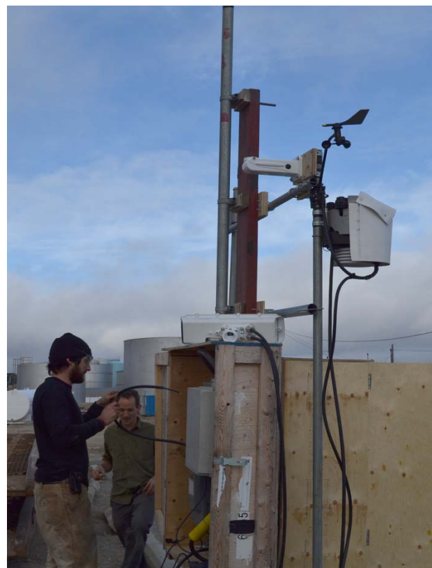
Fig. 5. The relay station in the process of assembly at Cambridge Bay dock.
