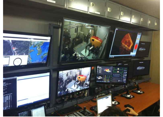
Fig. 4 Control and monitoring system of CR200.
