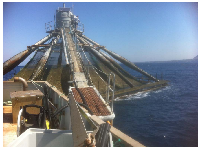
Fig.10 The mooring site of the buoy
