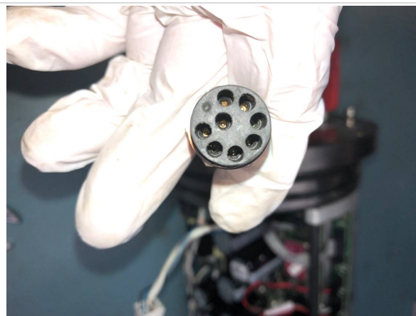
Picture # 2 Corrosion and damage found on TX connector
