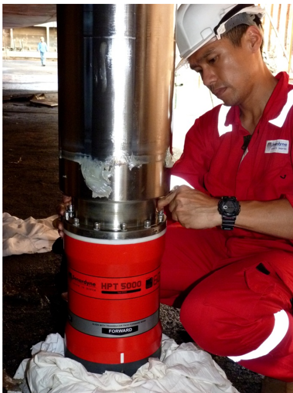
Figure 10–2 – Transceiver Lowered above Protective Material
