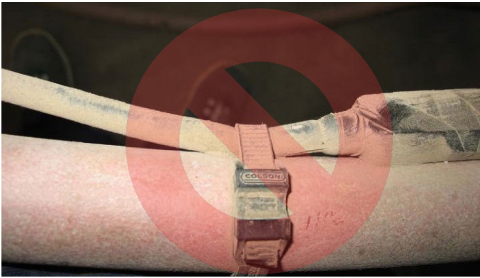
Figure 13. Do not use Zip-Ties Directly on Cables
