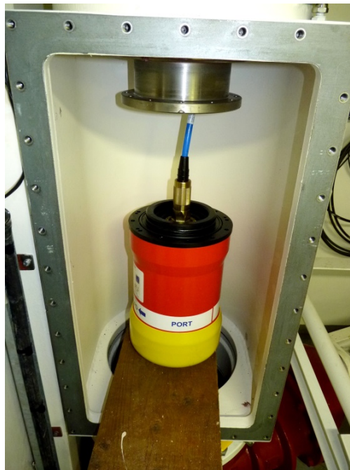
Figure 4-10 USBL Transceiver Cable Location
