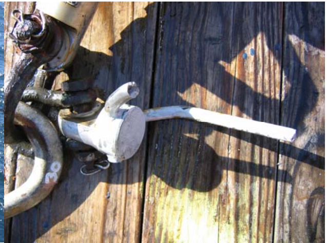
Figure 3. Load cell to release connection showing release cage failure.
