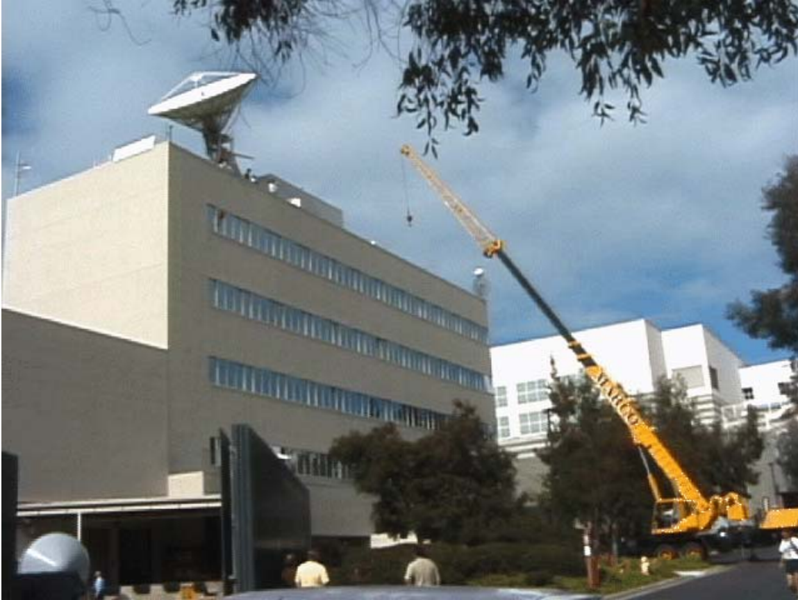
Figure 20: Shore-side Teleport hub antenna. By using a single, shared 7m class Earth station at the Teleport, 2.4m antennae can be used on the buoys. This minimization of buoy antenna size is critical due to the more difficult physical environment, requiring specialized motorization and tracking equipment.
