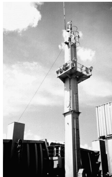
SeaLand ENTERPRISE and Bow Mast with IMET Modules at top.
