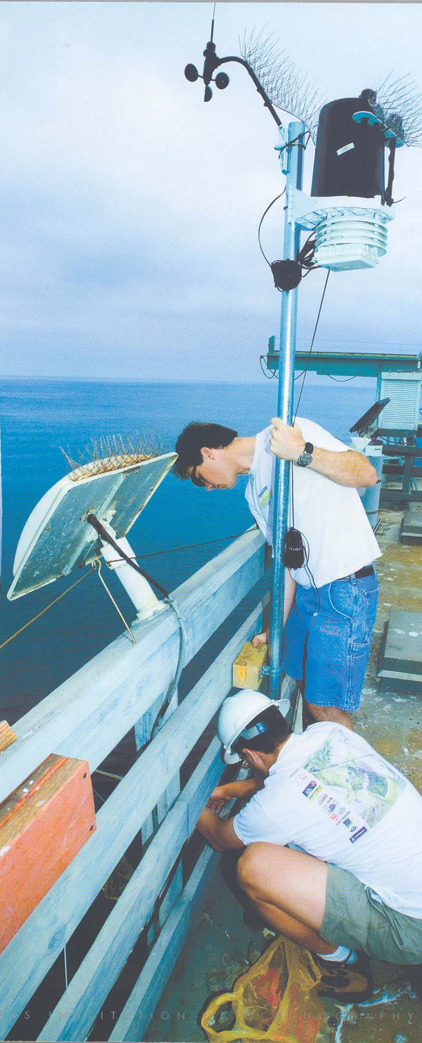
ROADNet technician Steve Foley carries a meteorological station assembled on an aluminum pole out to the end of Scripps Pier where he and technician Todd Hansen mount it on the roof of the pier shack.
