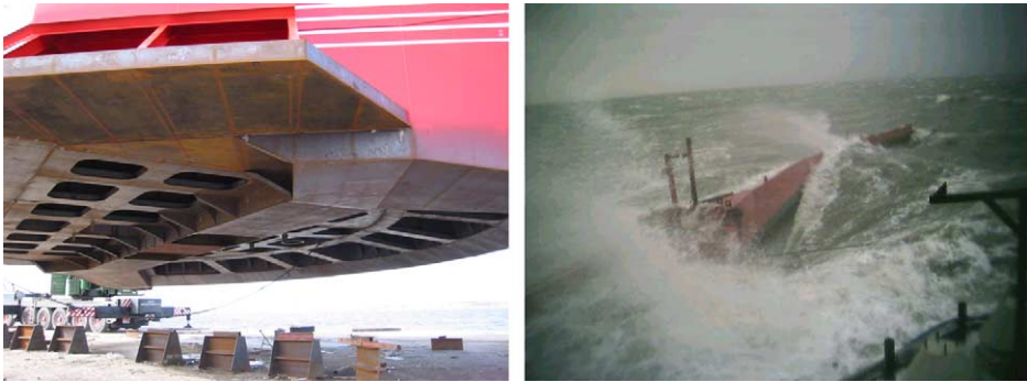
Fig. 4. Left : WD prototype at launch in March 2003. The open air-chambers are used to control the floating level. Right : WD prototype in heavy wave conditions.
