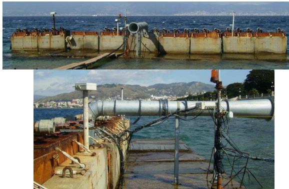
Figure 2 .- Pictures of breakwater and duct hosting the Wells turbine.
