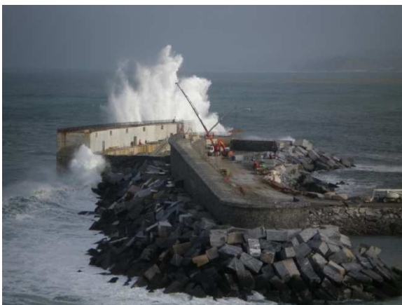
Figure 19: Construction of the turbine gallery
