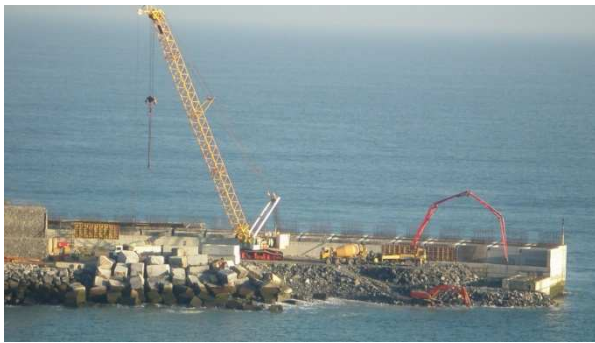
Figure 18. Covering the columns
