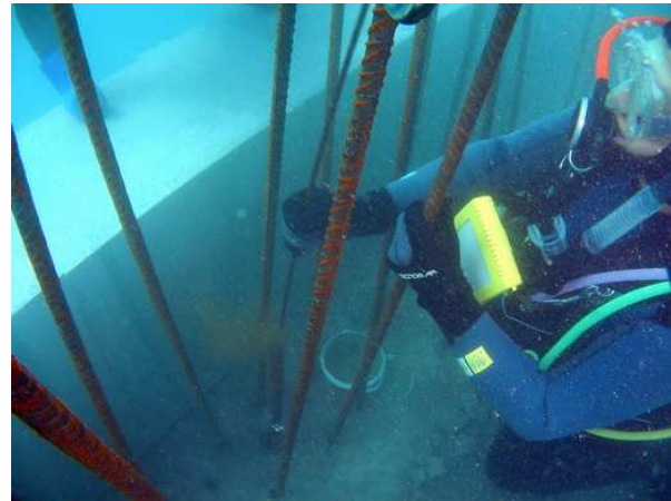
Figure 11. Undersea foundation works.
