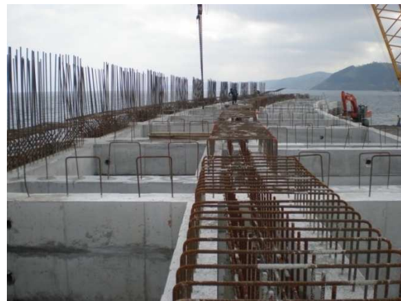
Figure 16. Columns before closure
