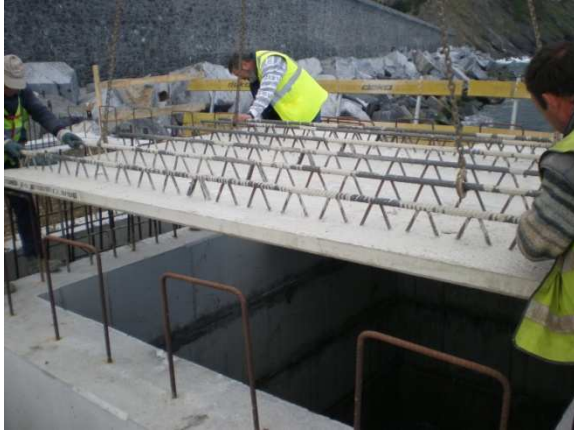
Figure 17. Layout of the permanent framework
