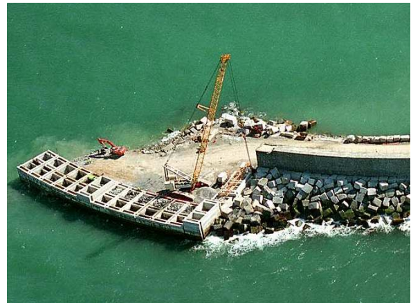
Figure 15. Power plant and breakwater joined
