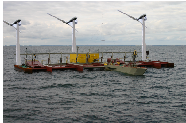
Figure 1: Picture of the Poseidon wave energy conversion platform at the test site at sea. The turbines are manipulated into the picture to show how they are suppose to be positioned.
