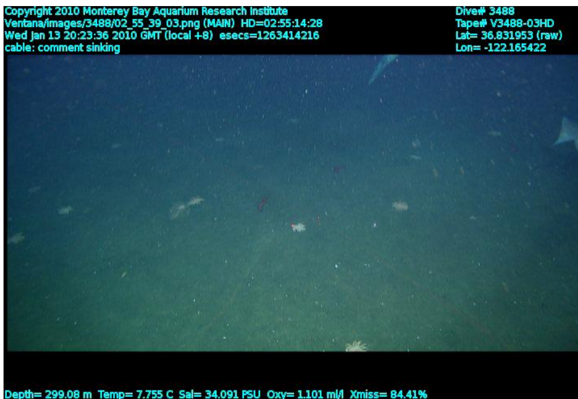
Figure 5. The cable is not buried along the neck of Smooth Ridge. In many sections, the cable is on the seafloor and sinking into the mud.
