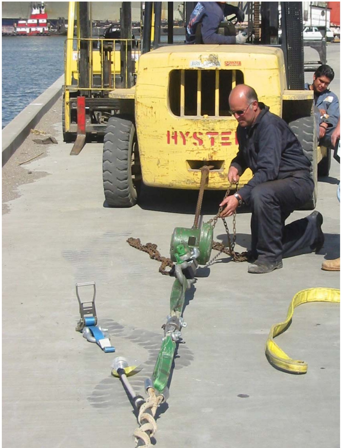
Load applied to remote cable end using pulley block and fork lift as dead man anchor
