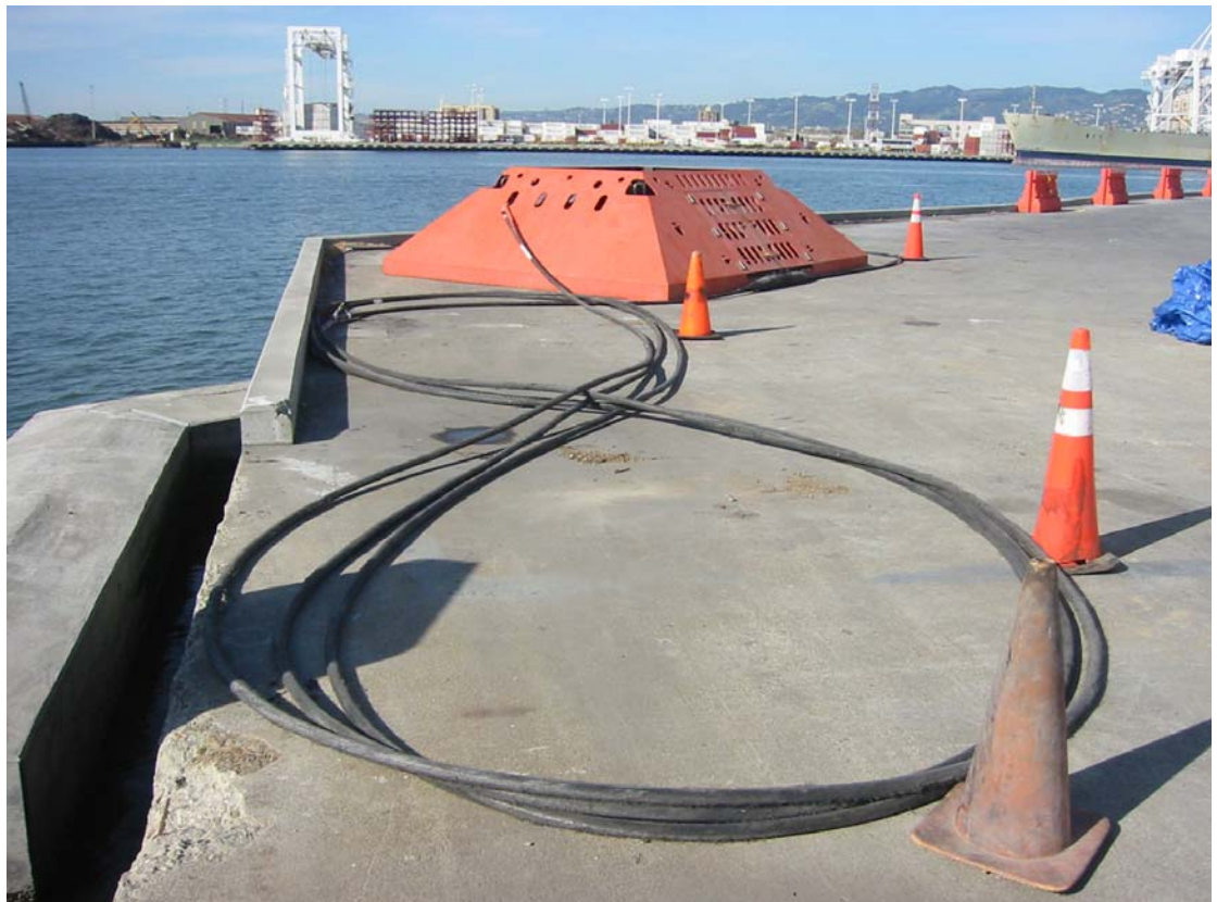
Cable stored on dock side in figure 8 on completion of tests.
