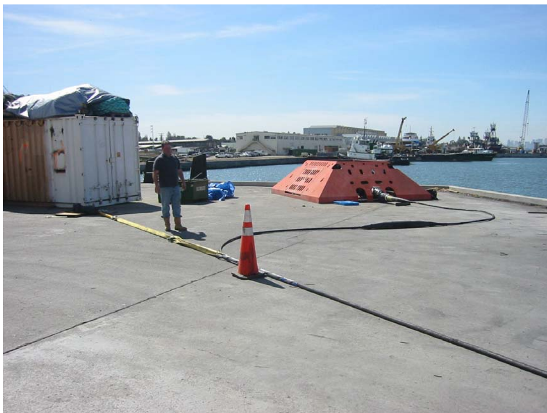
Cable secured to 40' container via preformed stopper outboard of anode joint.
