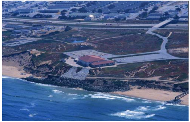
Fig. 16 Passive erosion in Central Monterey Bay due to placement of riprap.
