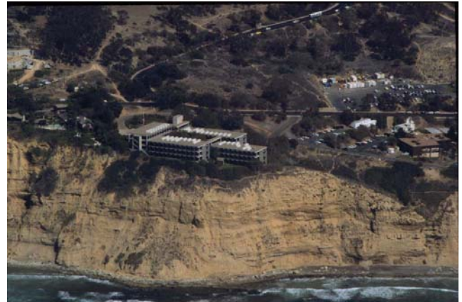
Fig. 11 National Marine Fisheries Service Building perched precariously on steep cliff in La Jolla.
