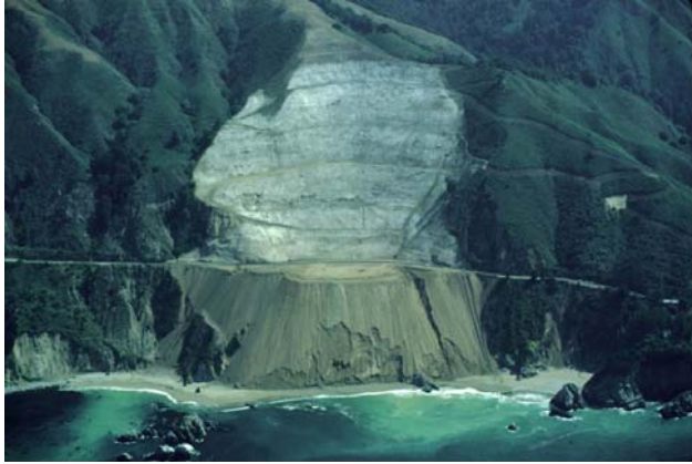
Fig. 4 Large landslide repair along Big Sur coast.
