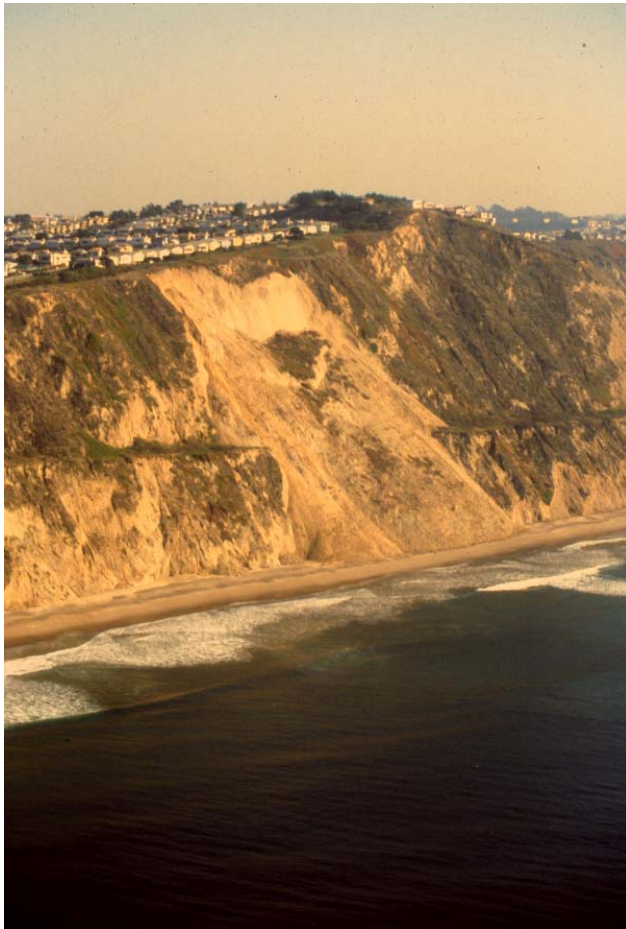
Fig. 10 Seismically induced bluff failure at Daly City, 1989 Loma Prieta Earthquake.
