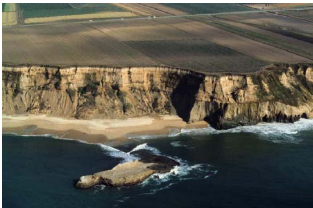
Fig. 2 Marine terrace and eroding cliffs in San Mateo County.
