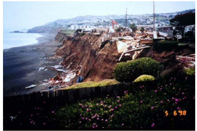
Fig. 14 1997-98 El Niño failure at Pacifica that led to loss of homes.
