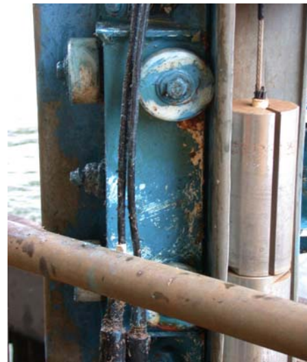
Fig. 6 Transducer carriage and support structure
