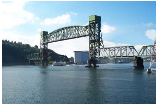
Fig. 4 Second Narrows rail bridge
