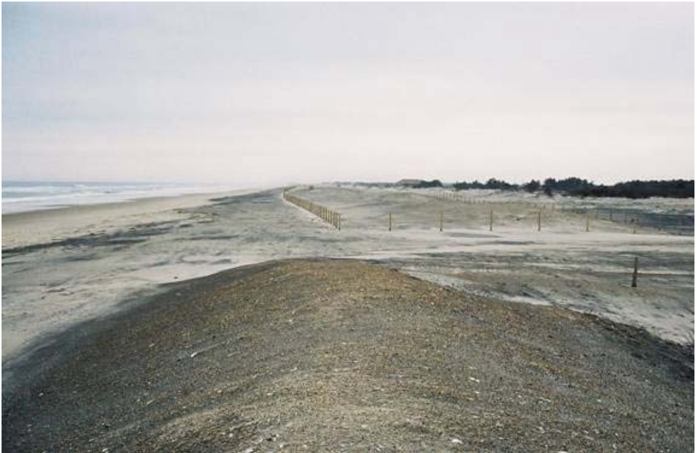
Figure 3. The berm along the northern portion of Assateague Island constructed using Federal OCS sand in 2002. The view shown in this April 2003 photo is toward the south.
