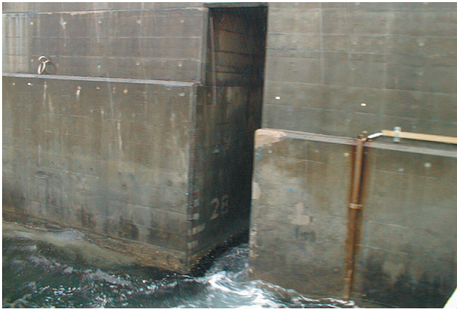
Fig. 14. Slit between caissons.
