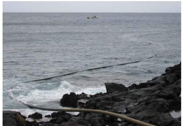
Figure 9. Deploying Borehole Liner Over Rock.
