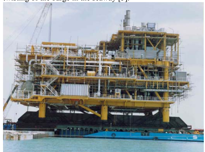
Fig. 14. Side view of Load out operation of SPP1 topside on SADRA FLB 124 barge.
