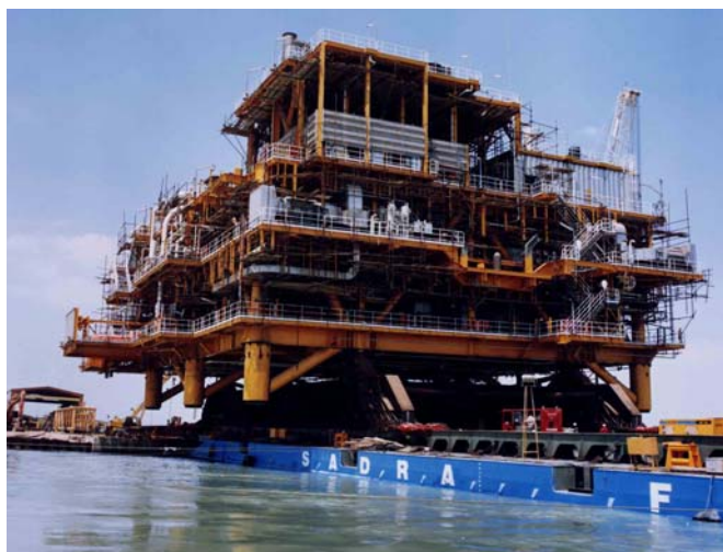
Fig. 15. Load out operation of SPP1 topside on SADRA FLB-124 barge.
