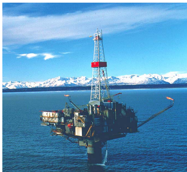
Fig. 1. A minimum facilities platform ( http://www.oilandgasreporter.com/ ).
