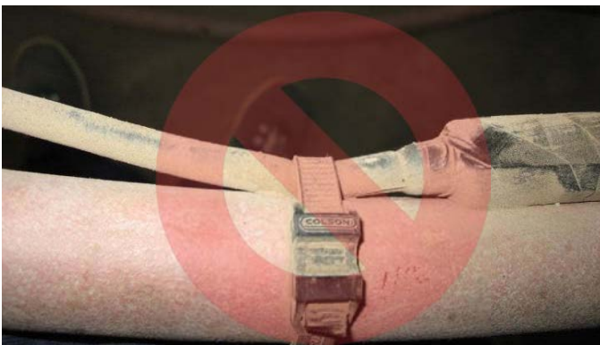
Figure 22. Do not use Zip-Ties Directly on Cables
