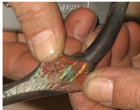
Figure 22. Do not use Zip-Ties Directly on Cables
