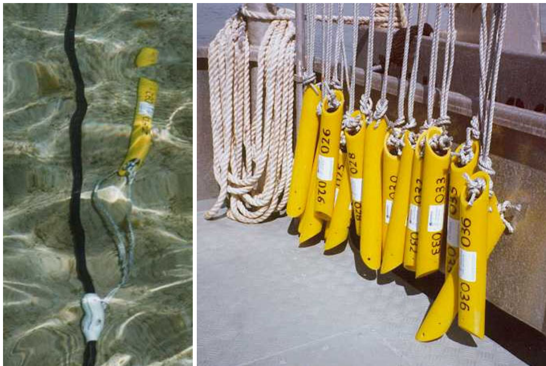
Transponders temporarily 'looped' onto the fixing point as the cable is deployed.
