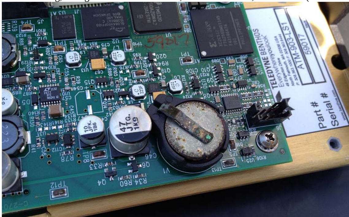
Coin cell on acoustic board stack has some surface corrosion/ discoloration. Cell removed for board cleaning, voltage measured at 2.997 V , model CVR1632; 3V nominal (= functional).
