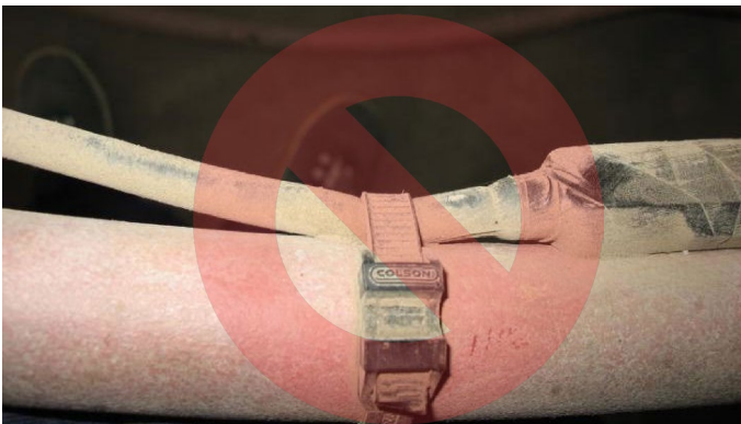
Figure 20. Do not use Zip-Ties Directly on Cables
