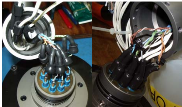
Fig 3: Close-up of connector during the assembly process
