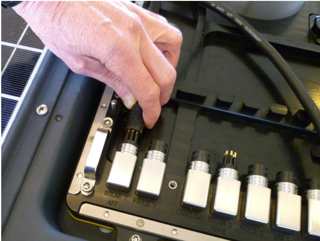
Figure 9.40. Attaching a Solar Panel Connector
