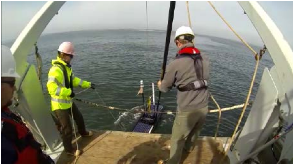
Figure 9.22. Hoist Line is Attached to Lifting Bail
