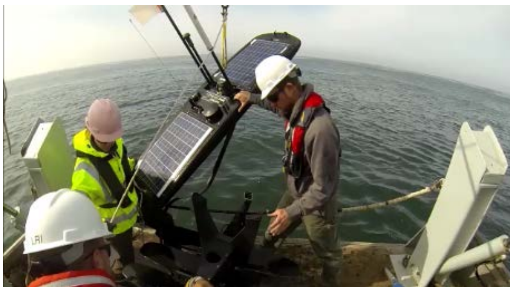
Figure 9.29. Placing the Saddle on the Sub
