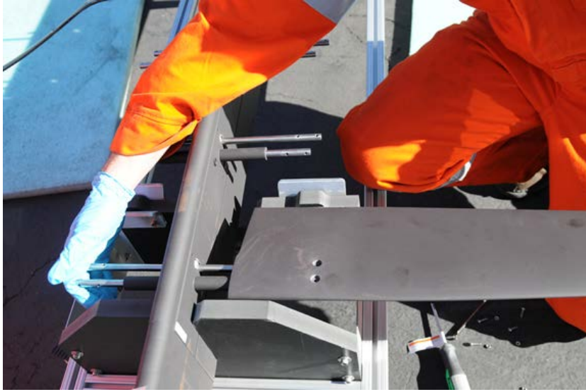
Figure 6.6. Sliding a Wing onto the Pivot and Spring Shafts
