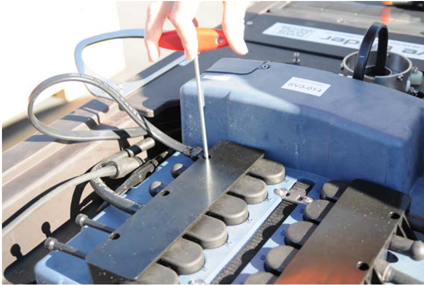
Figure 9.23. Install the Cable Bridge
