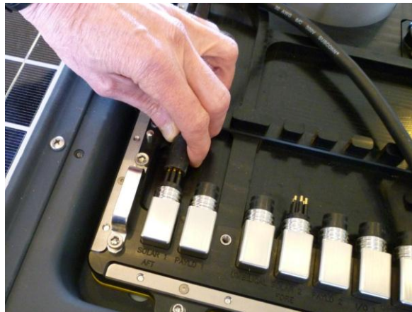
Figure 4-40: Attaching a Solar Panel Connector
