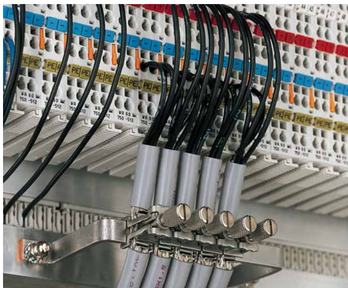
Figure 20: Application of the WAGO Shield Connecting System
