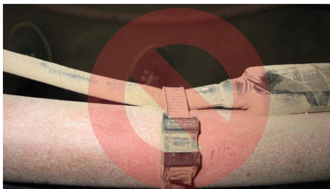
Figure 21. Do not use Zip-Ties Directly on Cables
