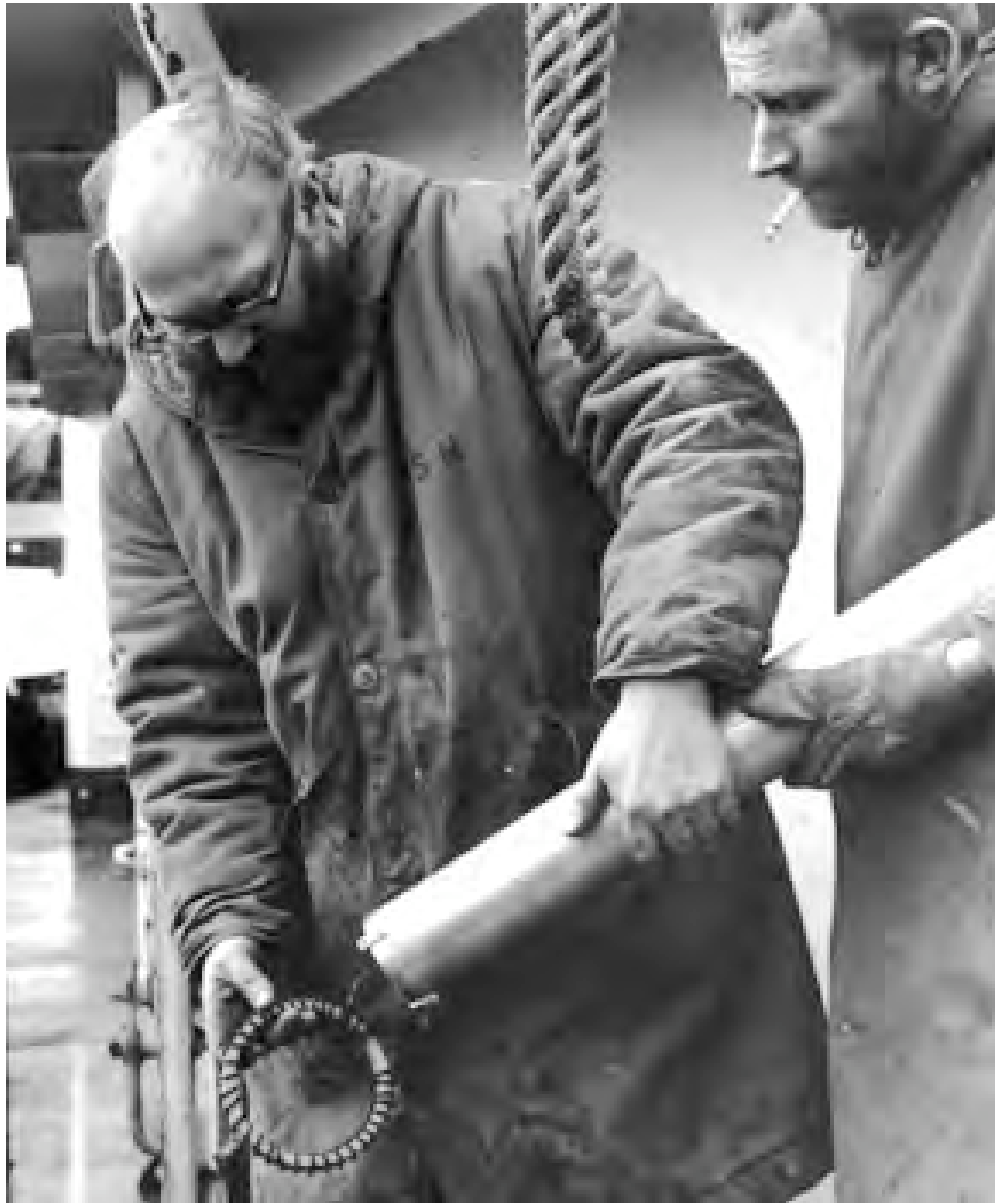
2) John Swallow (left) and Gordon Volkmann on R/V Erika Dan in 1962. The float shown here is essentially identical to floats deployed between 1957 and 1970 and using 10kHz magnetostrictive nickel scroll transducers. (Woods Hole Oceanographic Institution Archives)
