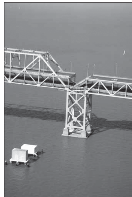
A section of the San Francisco-Oakland Bay Bridge collapsed in the Loma Prieta earthquake that occurred on October 17, 1989. So also did the double-decker portions of Interstate 880.
