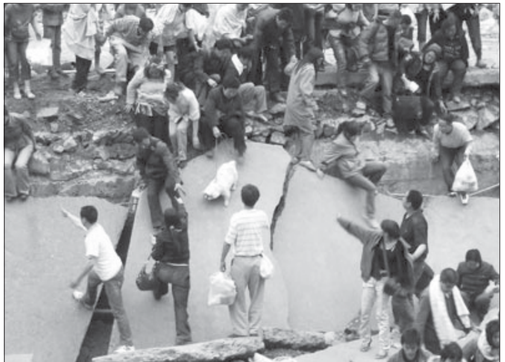
The earthquake that took place in Sichuan Province, China, on May 13, 2008, did extensive damage to bridges.
