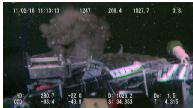
Fig. 7 Removing the Plug of Calcium Sulfate Minerals from top of tubing by ROV manipulator
