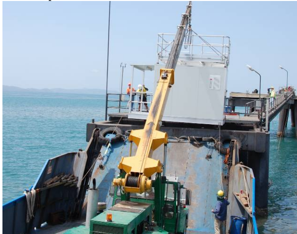
Figure 2. Installation of the instrument housing of observatory by crane on the 3 rd October 2009.
