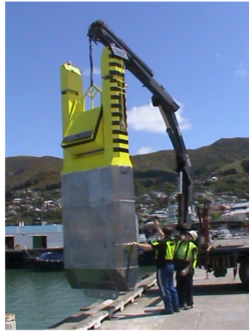
Fig. 5. The WET-NZ device being deployed at Lyttelton harbor
