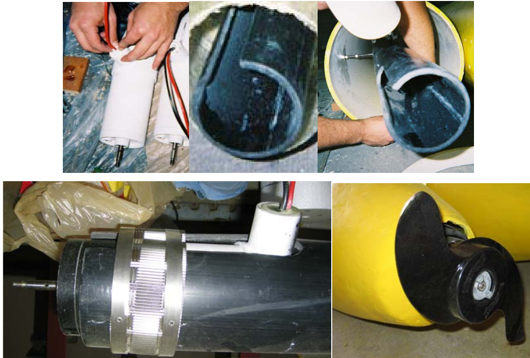
Figure 3.14 (a-e) From left to right, top to bottom: a) filling the cut shaft with epoxy, b) slot cut out from ABS for mounting thruster, c) bolts holding mounting in pontoon, d) thrusters mounted, and e) end cap mounted
