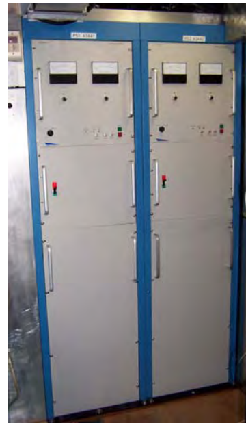
Figure 8. DTI COTS 200 kW, 20 kV power supplies.
