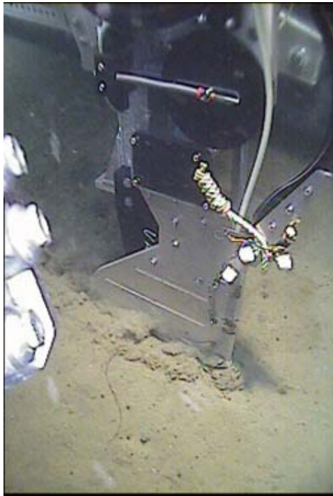
Figure 1: Laying the MOBB cable and burying it enroute
