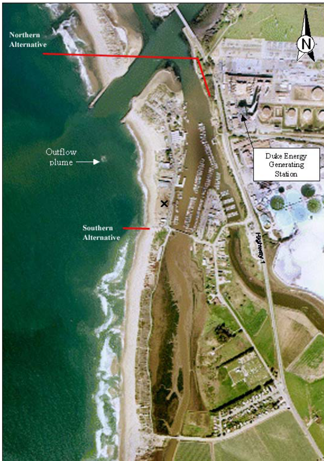
Figure 2-4 Existing Duke Energy Pipeline
