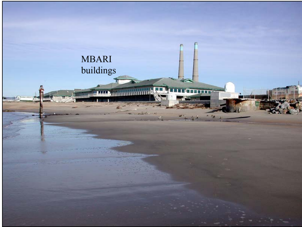
Photograph E-10 View northward at low tide across the proposed landing site (pier to be built) for the MARS cable.
