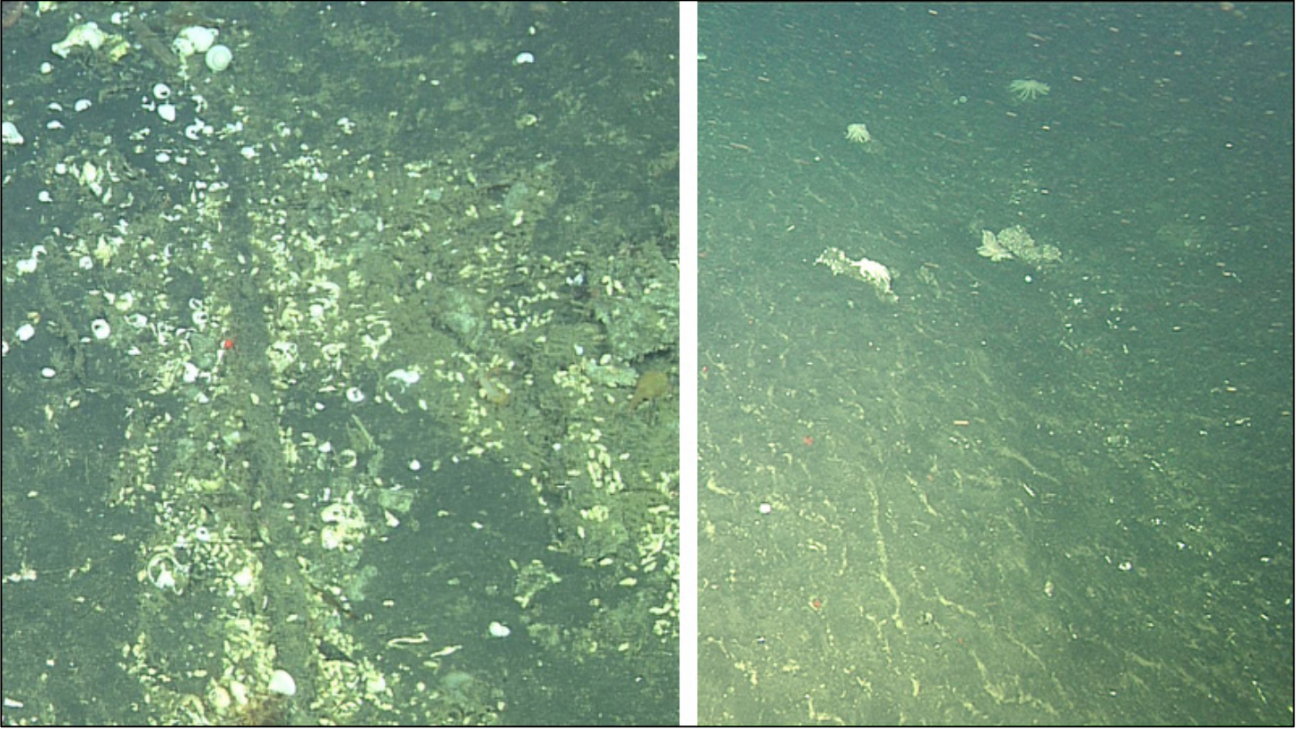
D. On Smooth Ridge, there are muddy areas where the surface-laid cable is now sinking into the sediment (left; 453 m water depth, D705, TC 05:31). The cable can no longer be seen in many places (right; 448 m, D705, TC 05:36).
